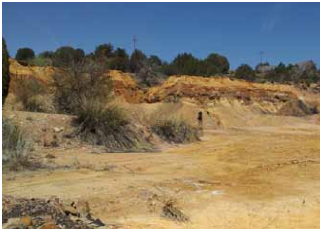
SAN VICENTE MILL SITE BEFORE REMEDIATION, INCLUDING REMOVAL OF SOIL AND WASTE PILES CONTAMINATED WITH HEAVY METALS. (GRIP PHOTO)
