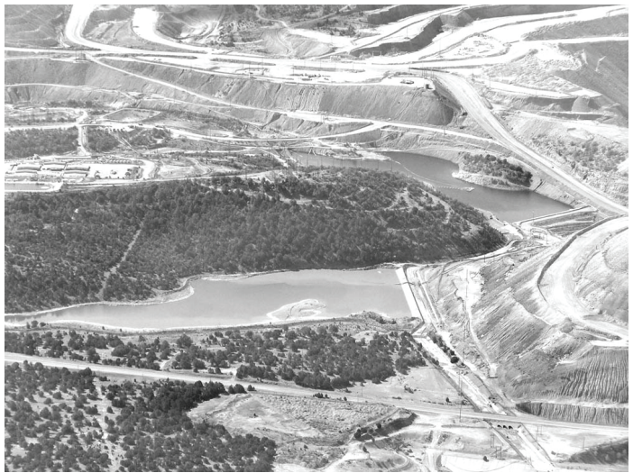
THOUSANDS OF GALLONS OF WASTEWATER ARE IMPOUNDED AT GRANT COUNTY MINES OWNED AND OPERATED BY FREEPORT-McMoRAN COPPER AND GOLD, WHICH HAS PROFESSED ITS COMMITMENT TO "SUSTAINABLE DEVELOPMENT" IN MANY CORPORATE DOCUMENTS. BUT DO ITS RECENT ACTIONS THREATEN OUR CURRENT AND FUTURE WATER SUPPLY? (GRIP PHOTO)
